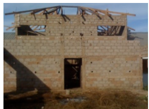
Conference Room with atrium's roof behind
